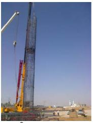
O-cell® cage lifting during installation
